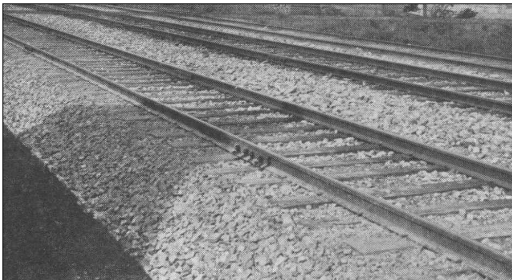
Figure 7. Tracks over typical stone ballast (Howson 1926:146)
