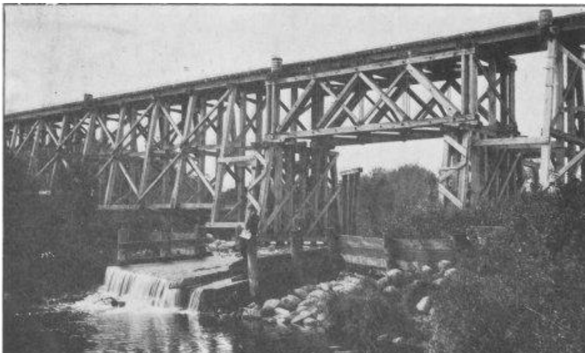
Figure 16. Great Northern trestle at Mayville, ca. 1900 (State Historical Society of North Dakota, A4405)
