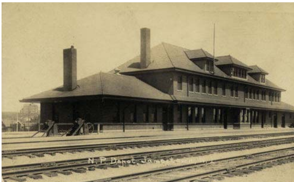
Figure 4. Multiple Tracks at Jamestown Railroad Station, ca. 1910 (Institute for Regional Studies, North Dakota State University, 2000.263.86)
